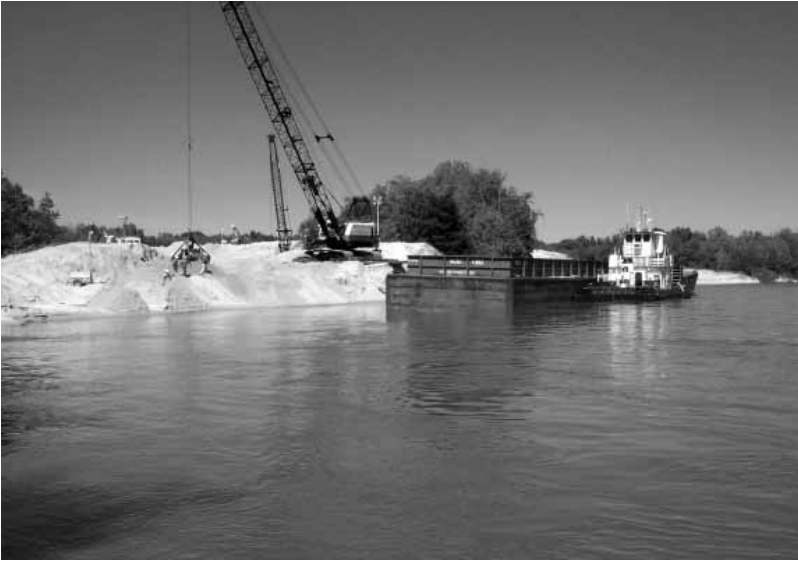
Fig. 3.4b. The U.S. Army Corps of Engineers transfers sand from spoil site 40 to replenish beaches. Photo by John Crowe.
